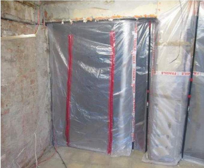
Secured and quarantined area for the Asbestos removal.
